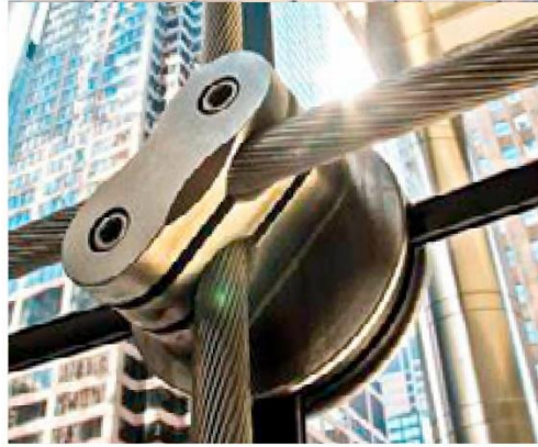
Single Cable Point-fixing Curtain Wall
