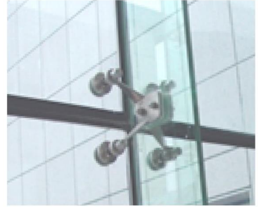
Glass Rib Supported Point-fixing Curtain Wall
