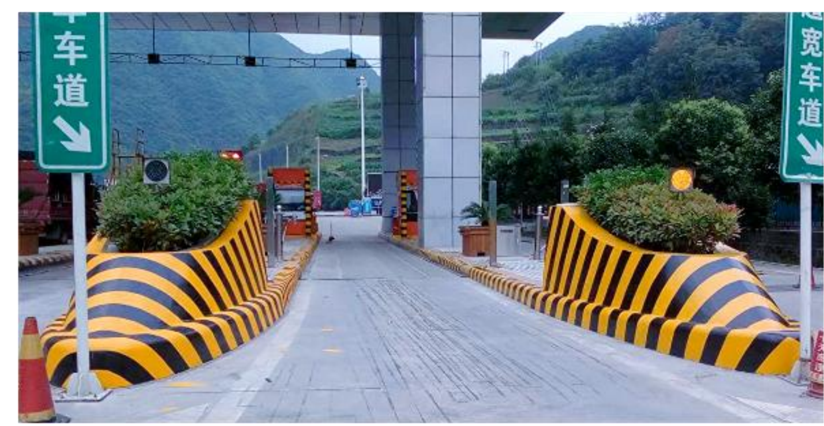
Toll island warning signs
