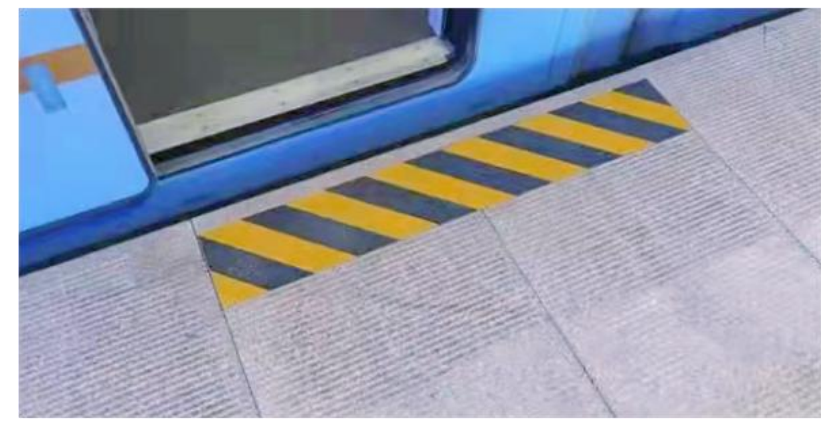
platform warning tape
