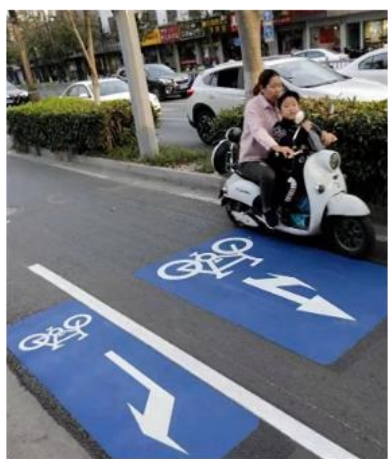
Ground Markings for Non-Motorized Vehicle Lanes
