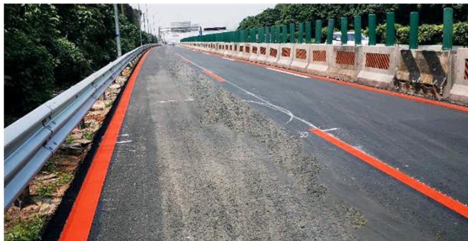
Temporary road markings for Guangzhou Expressway expansion and renovation
