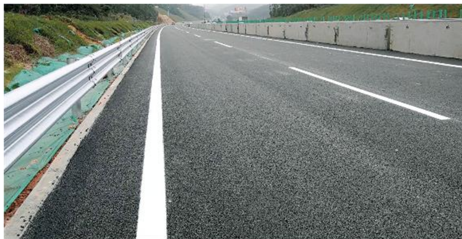
Temporary road markings for Shandong Expressway expansion and renovation
